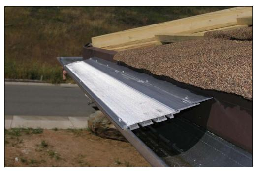
Gutterglove has been successfully installed on a 6 inch half round gutter.
