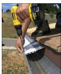
The final step is to install Gutterglove. There are no screws or support brackets holding up the back because Gutterglove rests on the fascia board. Because the front is screwed down tightly to the front lip of the gutter, the back cannot come up.
