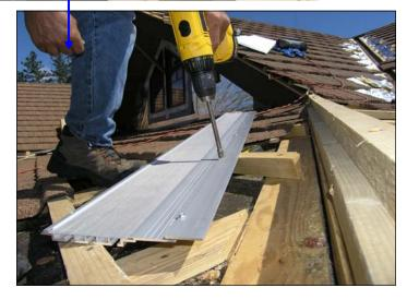
Screw down the strip to the back of Gutterglove. You may have to pre-drill first.
